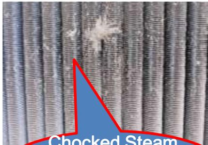
Chocked Steam heater coil attached with Hot air blower
