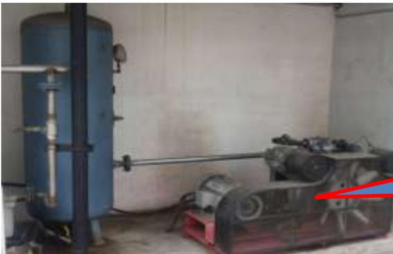
Replace inefficient reciprocating compressor, Reduce energy consumption and maintenance cost
