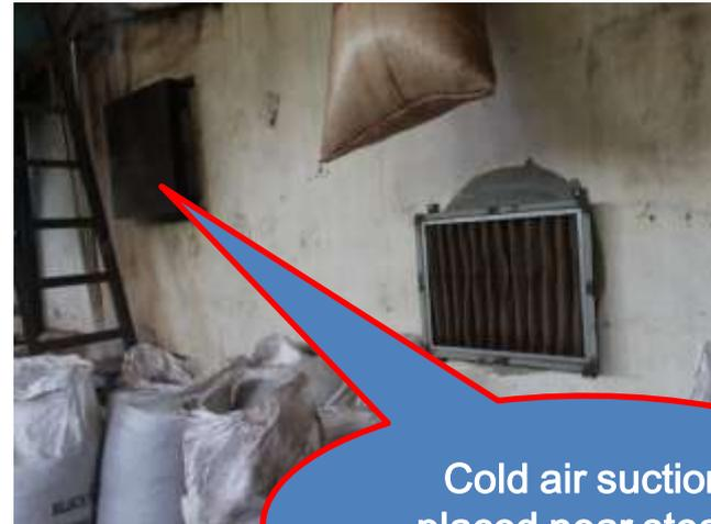
Cold air suction placed near steam trap and covered
